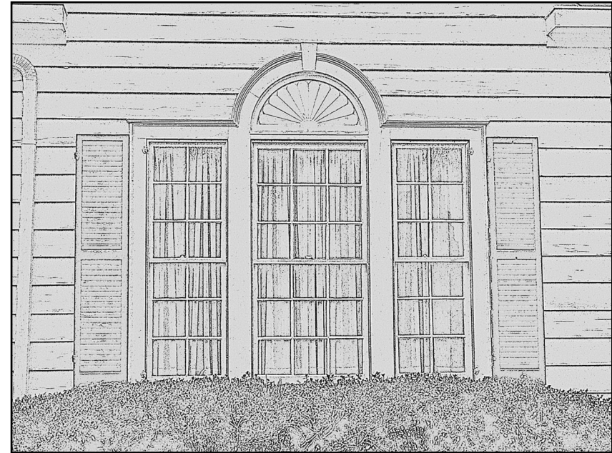
These decorative shutters are too small to serve their historic function.
