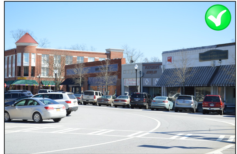
The roof of this mixed use structure (left) is predominantly flat like the historic buildings in the foreground. Covington Historic District
