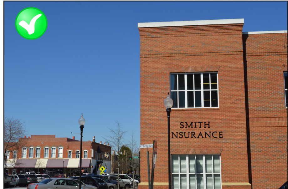
Materials on the newer commercial building (right) are similar to the historic commercial building on the left. The cornice is capped with metal, but painted white to lessen the metal's appearance. Covington Historic District
