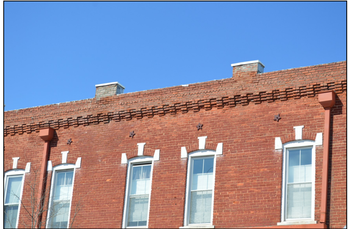
Here is an example of an intact corbelled brick cornice on a commercial building. Covington Historic District
