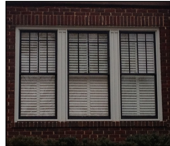
Intact true divided lights are integral to the historic character of this house. Covington Historic District
