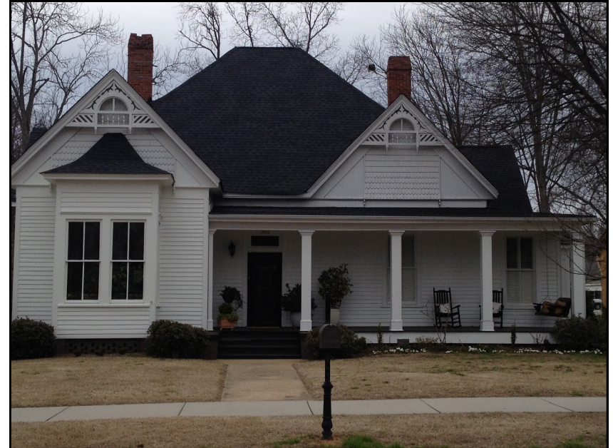
The porch is a significant feature of the facade. Covington Historic District
