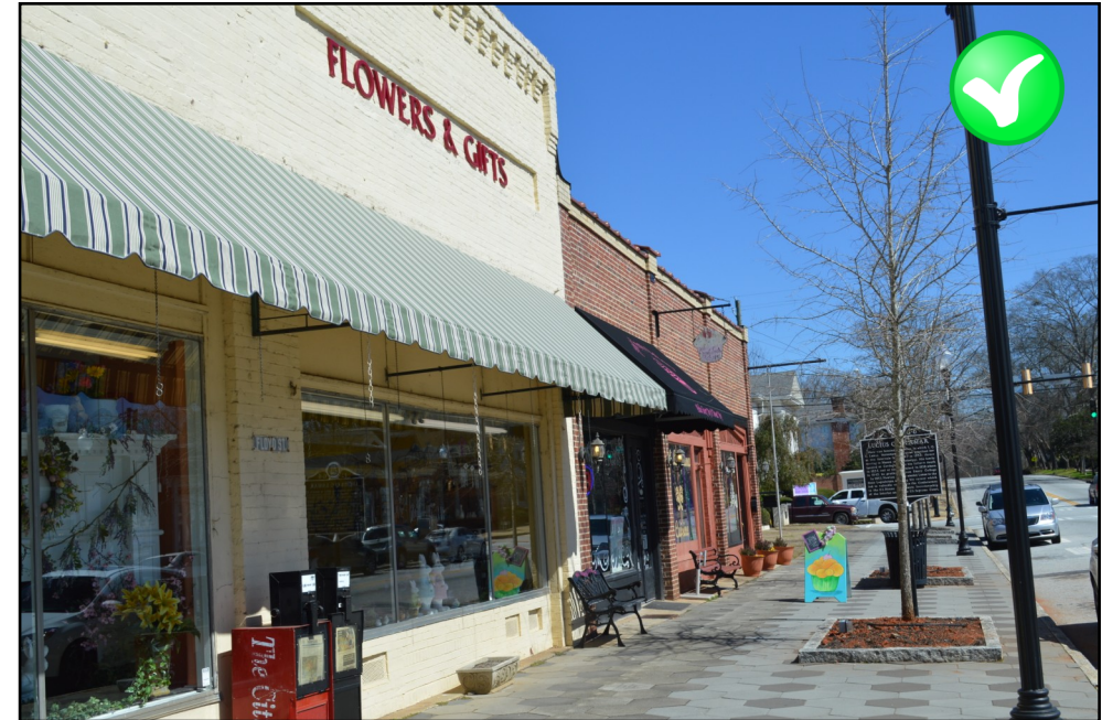
These commercial buildings along Floyd Street display appropriate fabric awnings with a scissor-cut valance. Covington Historic District
