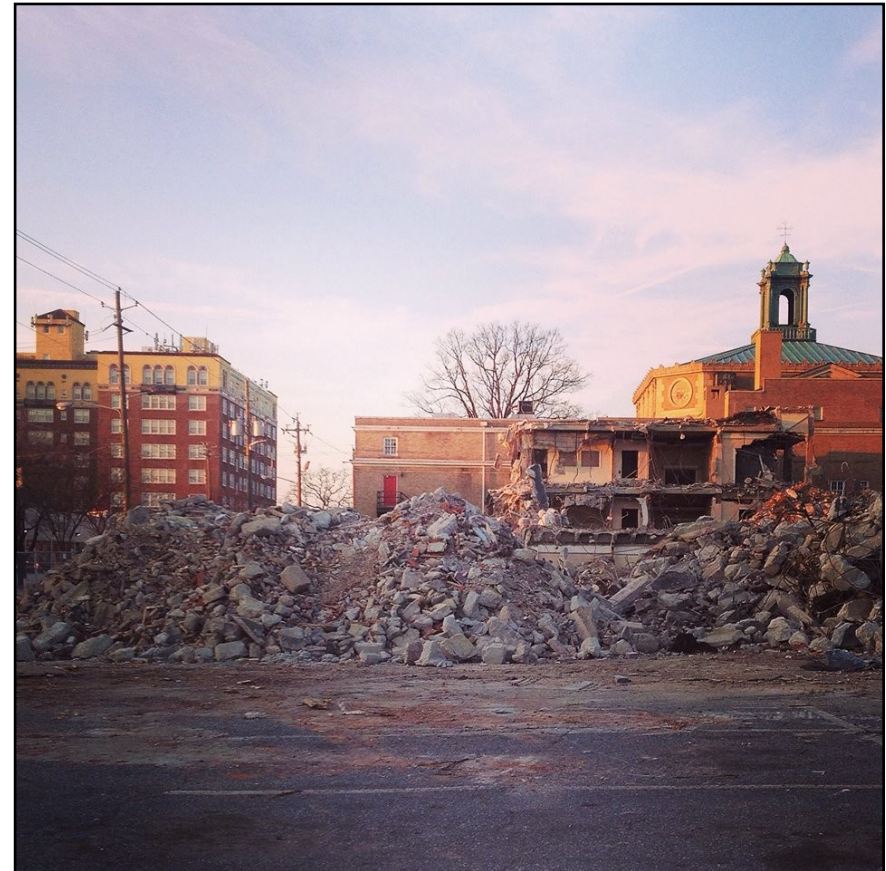
The demolition of this 1950s building in the Poncey-Highland neighborhood of Atlanta, though not in a district subject to design review, serves as an example of a lost historic resource.
