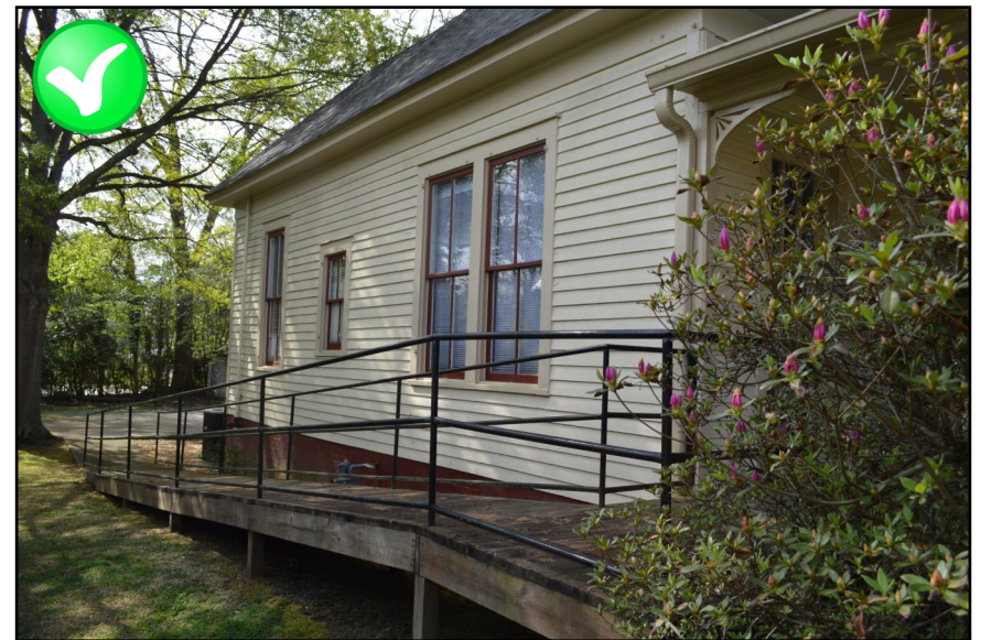
Appropriate example of an accessibility ramp integrated into a residential building with minimal alteration to the historic design and materials.
