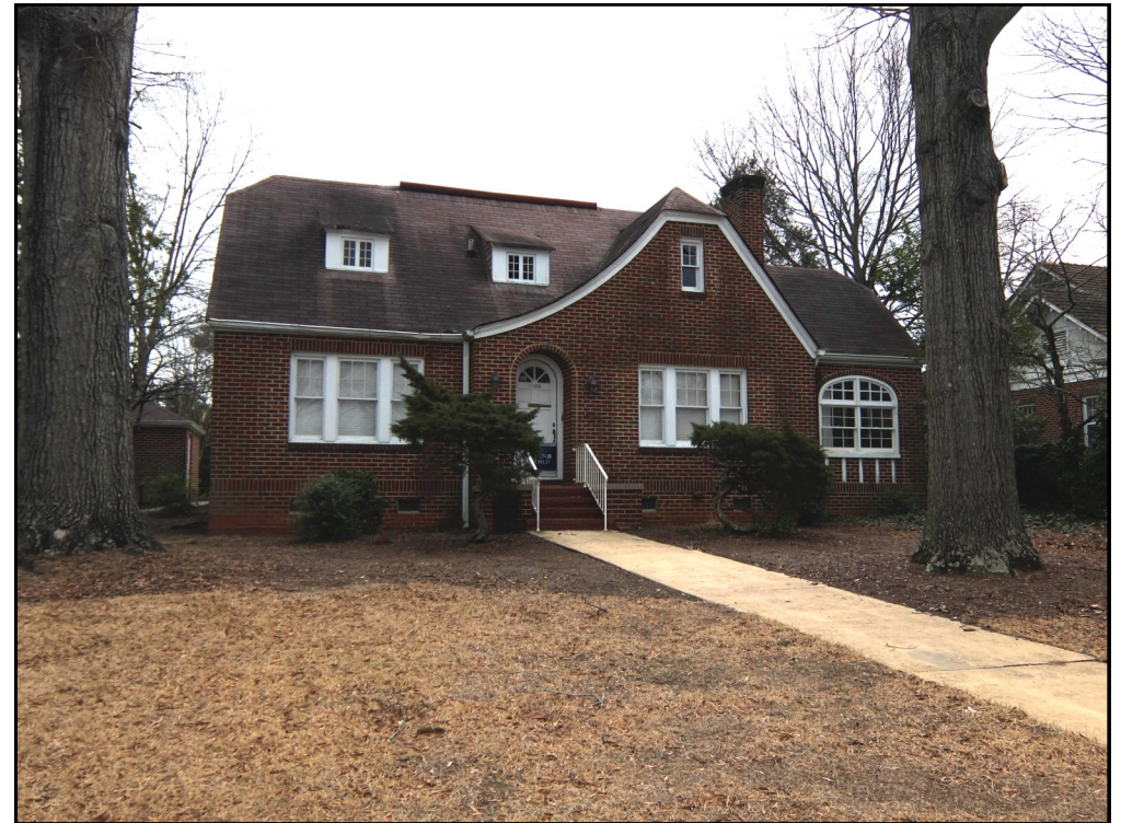
An example of an English Vernacular roofline. A sweeping gable with historic dormers and jerkin head gables combine to create this distinctive appearance. Covington Historic District
