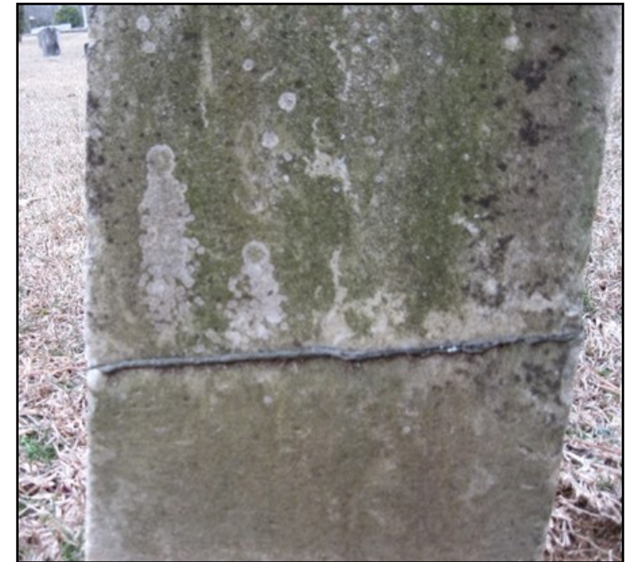
Photo 12: Inappropriate Repair Using Epoxy
