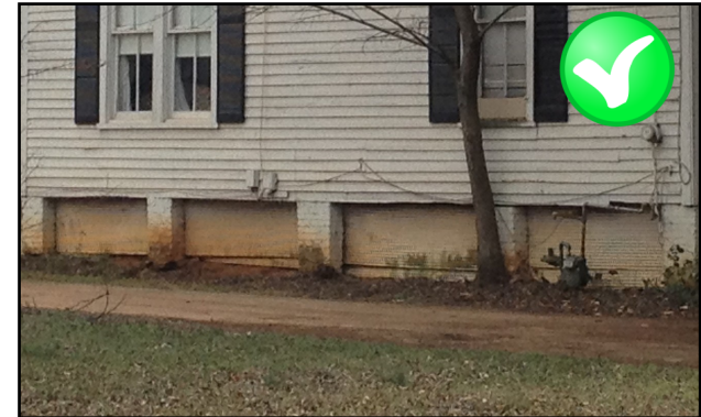
This foundation features an appropriate delineation between historic piers and new infill. North Covington Historic District
