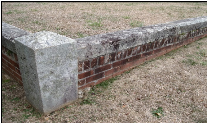
Photo 4: Brick Retaining Wall with Marble Corner Stones and Coping
