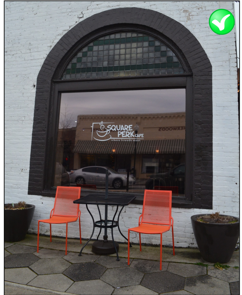
The brick work, frame, and transom of this ground floor arch window has been appropriately maintained. Covington Historic District.
