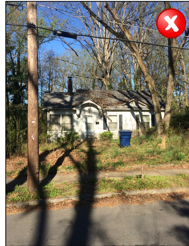
Improperly maintained buildings, such as this historic house, detract from the overall character of a historic district.
