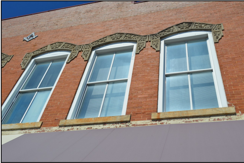
The decorative stonework around this window is integral to the building's character. Covington Historic District.
