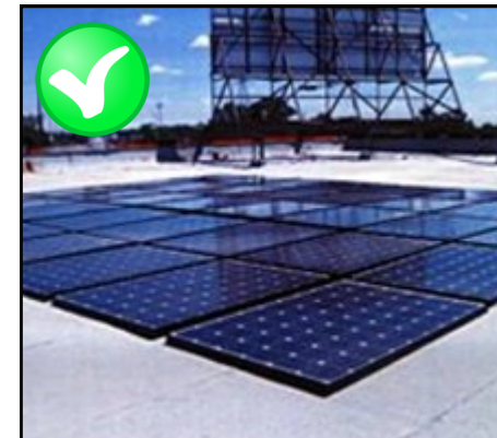
The solar panels on this historic building are flat and hidden behind a parapet wall, and thus out of the public view.
