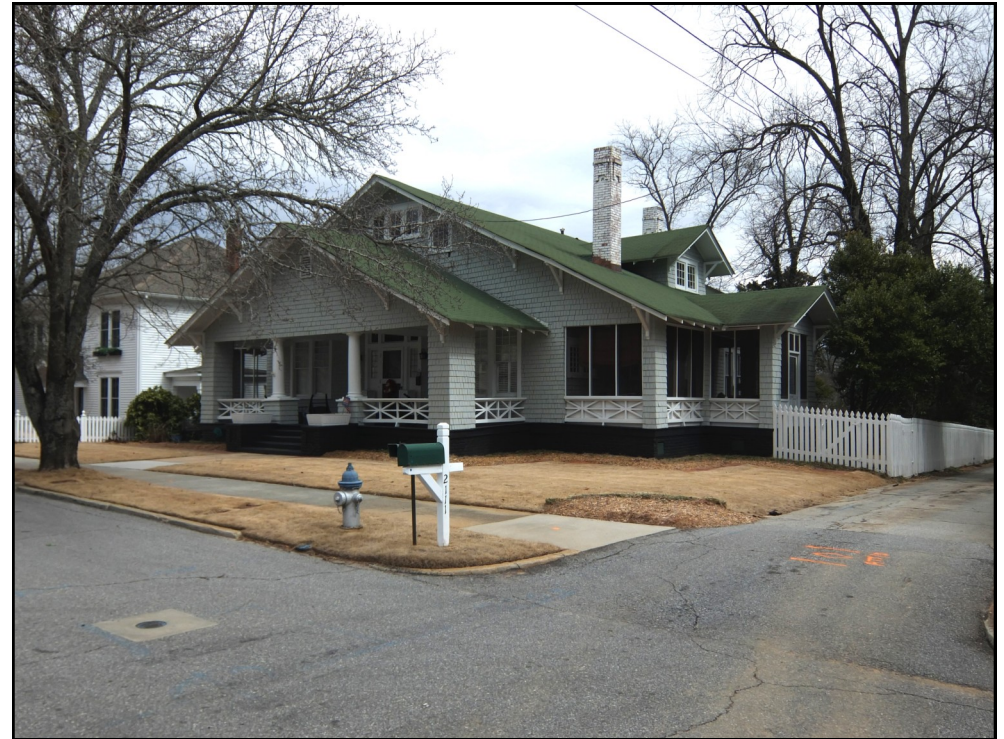
Historic shingle siding, large brackets, and chippendale railing all define this Craftsman Bungalow. Removal or change in material would detract from the historic integrity of this residence. Covington Historic District
