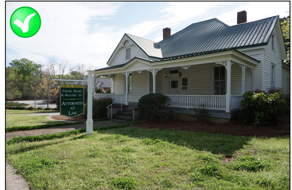
Appropriate example of historic house featuring stand-alone post and arm signage in the yard.
