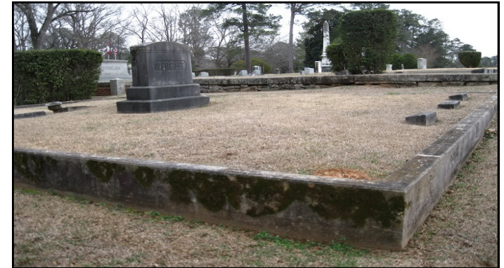
Photo 3: Concrete Retaining Walls
