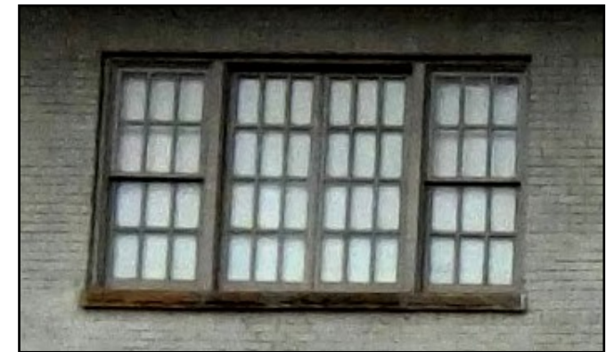
Tripartite windows with varying lights are character-defining to the façade. Covington Historic District
