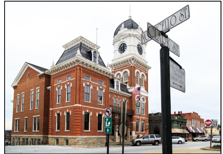
Newton County Courthouse. Covington Historic District
