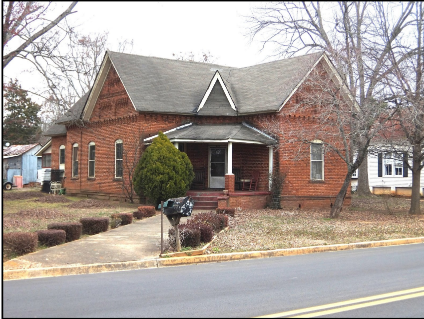
Cross gabled roof with projecting central gable and pent roof over porch are character-defining features of this house. Covington Historic District
