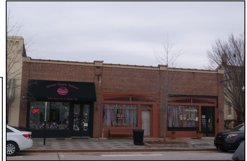
These storefronts along Floyd Street are common on commercial buildings in Covington. Covington Historic District.
